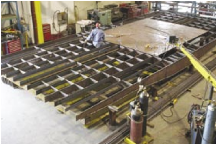
MAJOR FABRICATION Replacement ramp for car ferry.
