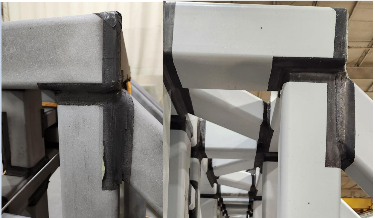
Figure 2: Taped off welds (before and after paint)
