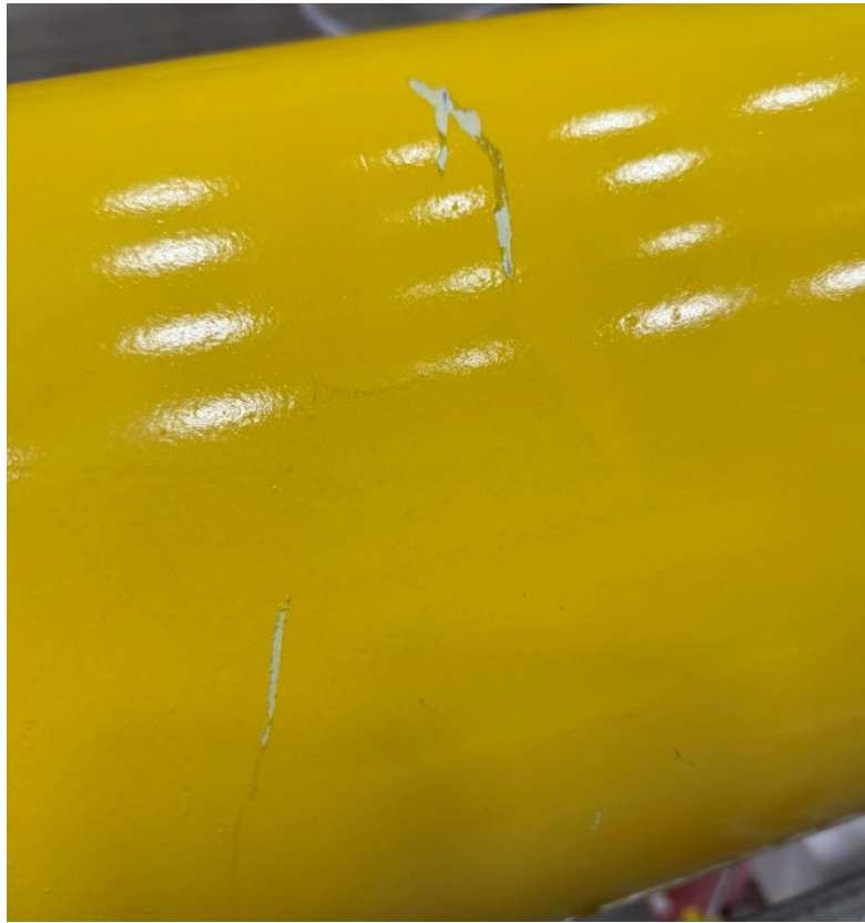
Figure 11: Unacceptable scratching and marring
